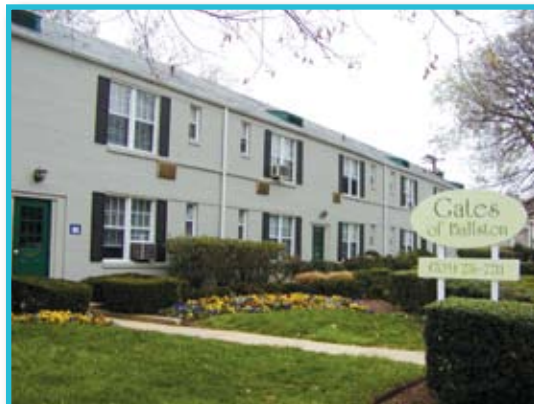
◀ AHC, Inc. development The Gates of Ballston a 464 unit mixed-income development.
